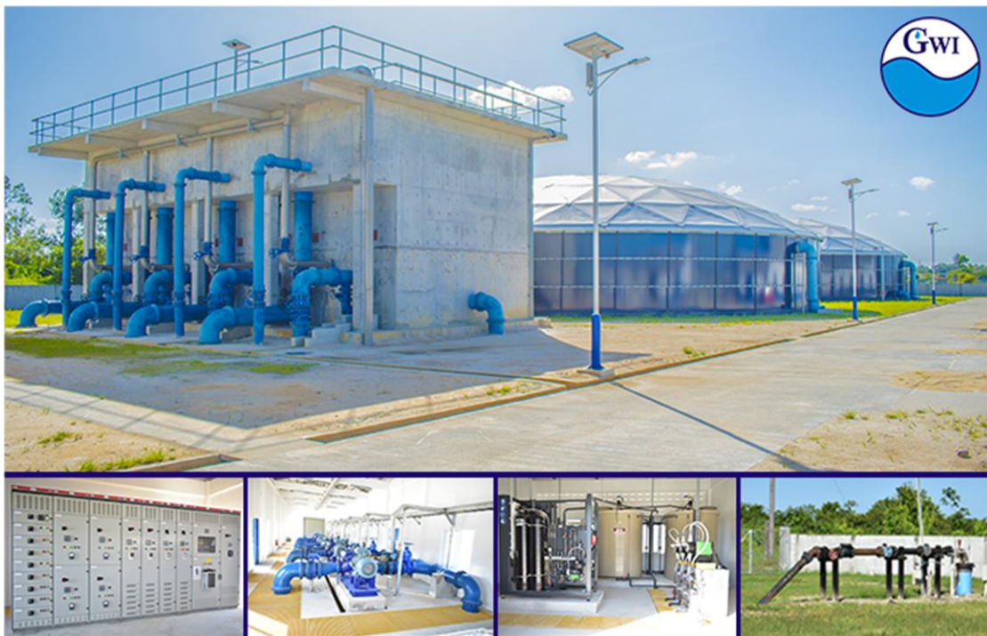
New Water Treatment Plant at Diamond, EBD
